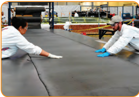
Carbon Fiber Lay-up
