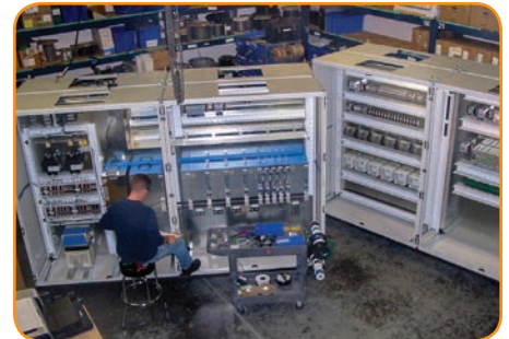
Janicki UL Cabinet Shop
