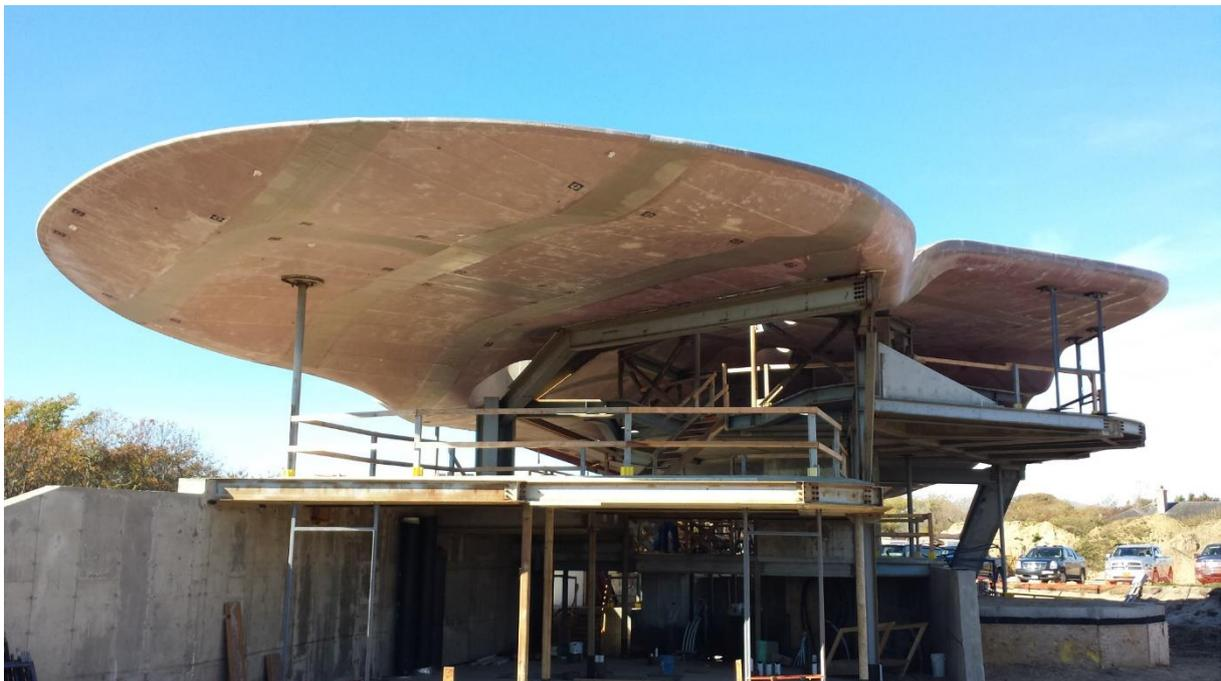
This innovative solution concerns a composite that is forming the finished inner and outer surfaces as well as the primary structure of a roof. The composite roof replaced nearly all the supporting steelwork with a self-supporting very thick FRP/foam cored sandwich structure.
