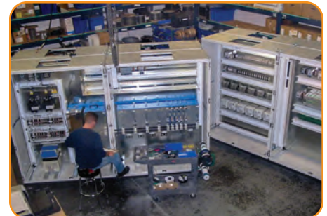
Janicki UL Cabinet Shop
